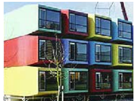
The sustainable buildings designed by ecosistema urbano are a series of 3D components.
