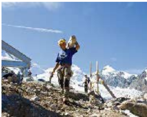
Splendid isolation on-site – workers return to the valley on weekends.
