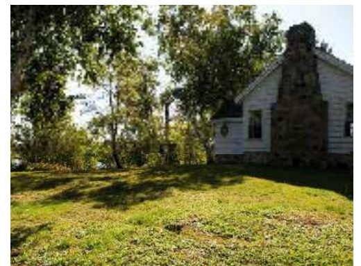
The internationally-renowned Cooperative Freshwater Ecology Unit currently calls four cottages home but the team’s needs have outgrown these simple structures.
