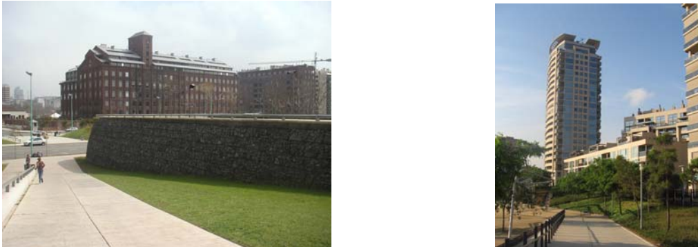
Figure 1: so called “public” parks sometimes feature “divisions” which end up segregating one class from another. Micaela Bastida Park, Puerto Madero, Buenos Aires and Diagonal Mar Park, Barcelona.
