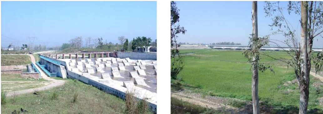
Figure 2.4a, 2.4b: The Upper Ganges Canal intersecting intermittent rivers, under and over
