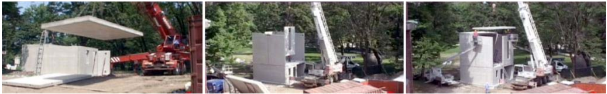
Figure 5: Prefab: Assembly Process
