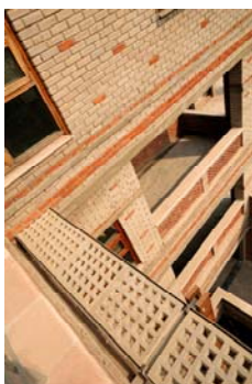
Figure 6: Earthen Construction of Dome: Satprem Maini www.auroville.org
