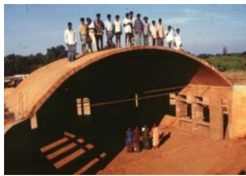
Figure 6: CEB construction: Ashok Lall
