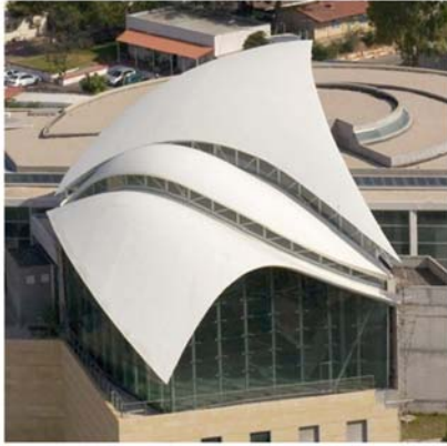
Figure 5: Yitzak Rabin Center Roof
