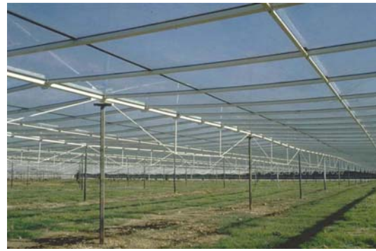
Figure 2: Solar updraft tower, glass greenhouse
