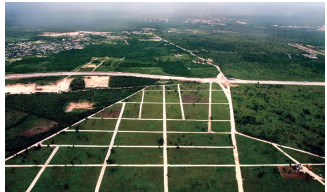
Fig. 2: Residential development in Veron, Higuey, Dominican Republic, and the new boulevard built by the Dominican government in association with private investors.
